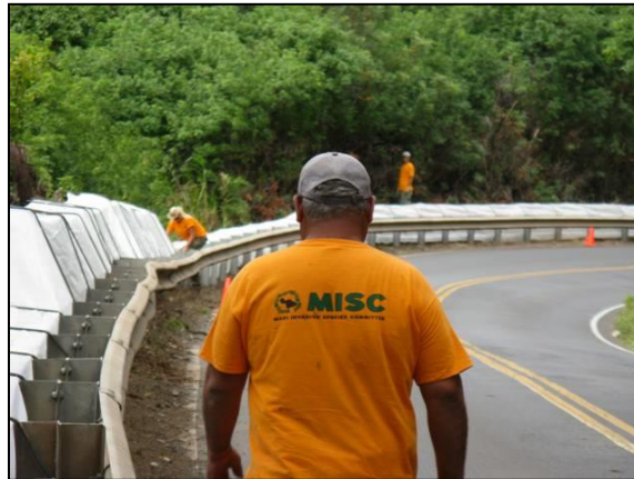
Figure 14. Barrier fence along Kaluanui Road
