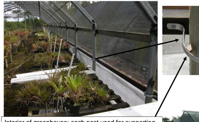
Interior of greenhouse; each post used for supporting wood located on the outside of greenhouse. Screen stapled to wood.
